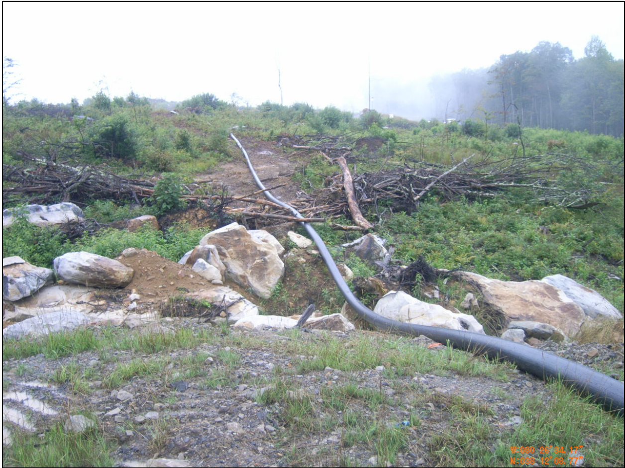
Figure 19: Unsupported Pipe at Plum Creek
