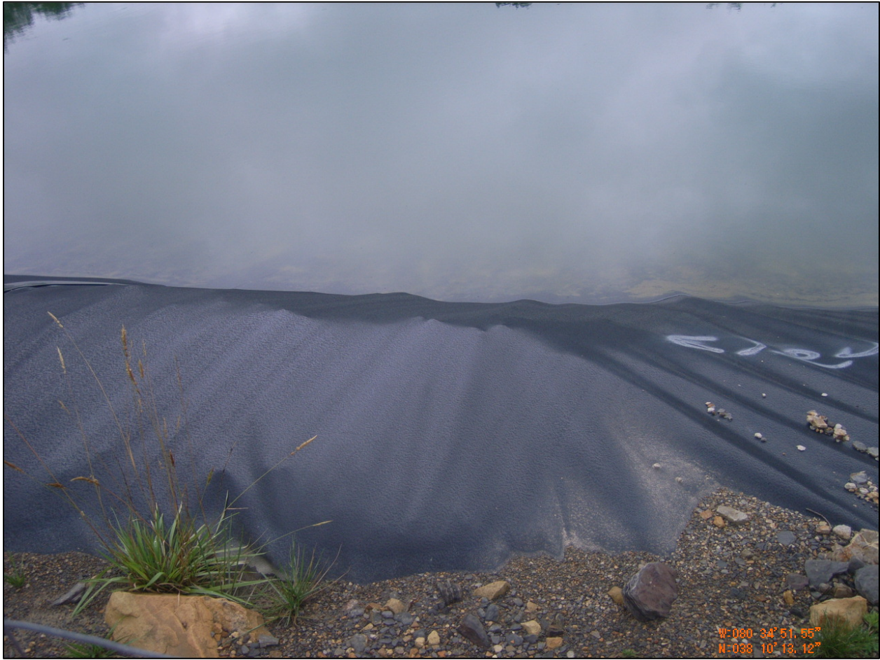
Figure 16: Liner Bulges at MWV
