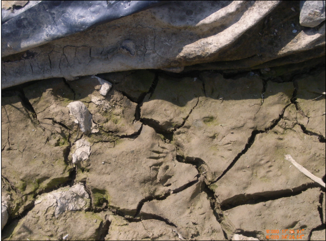
Figure 4: Settlement Cracks in Anchor Trench
