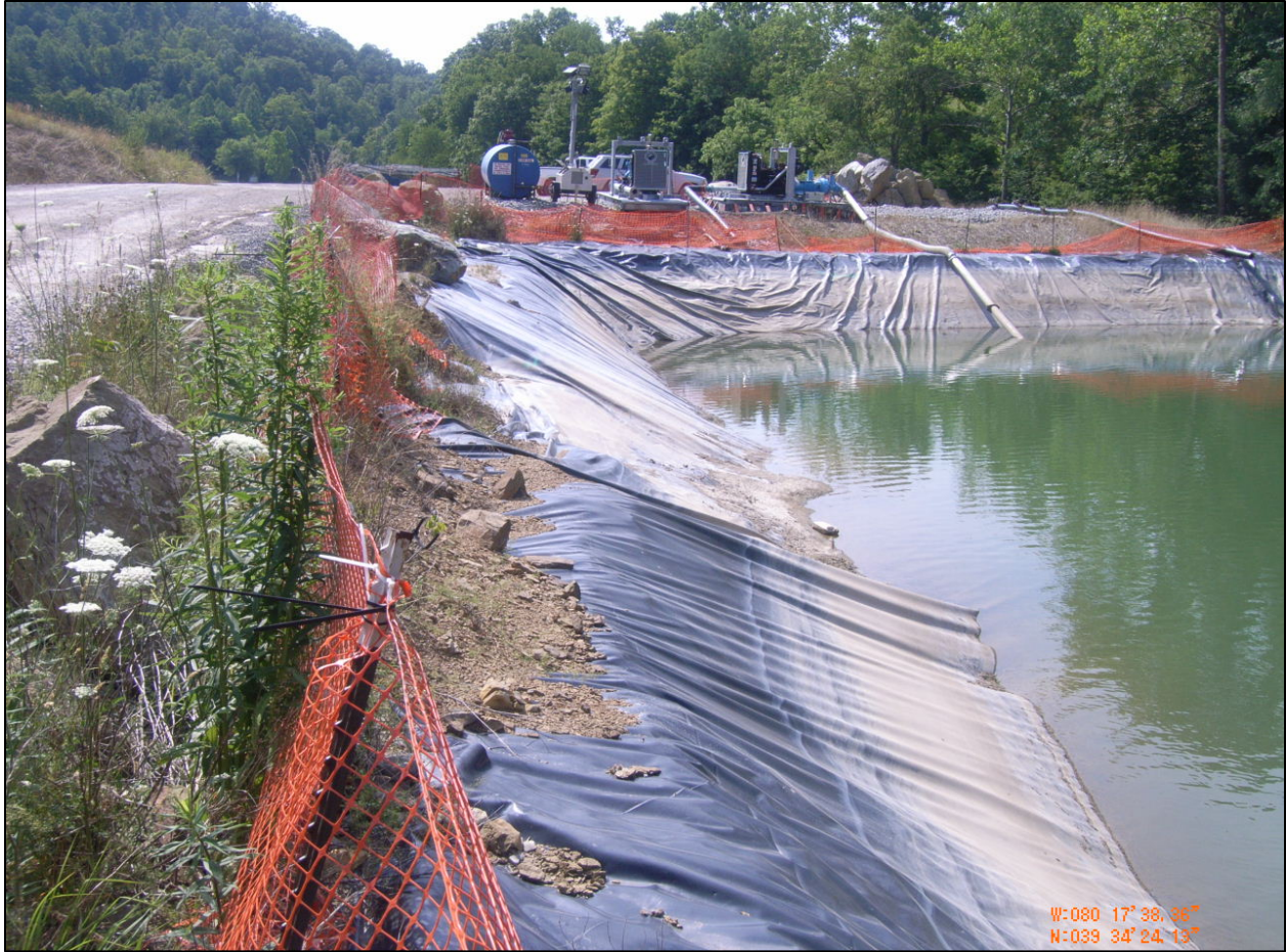
Figure 8: Rock and Debris on Liner
