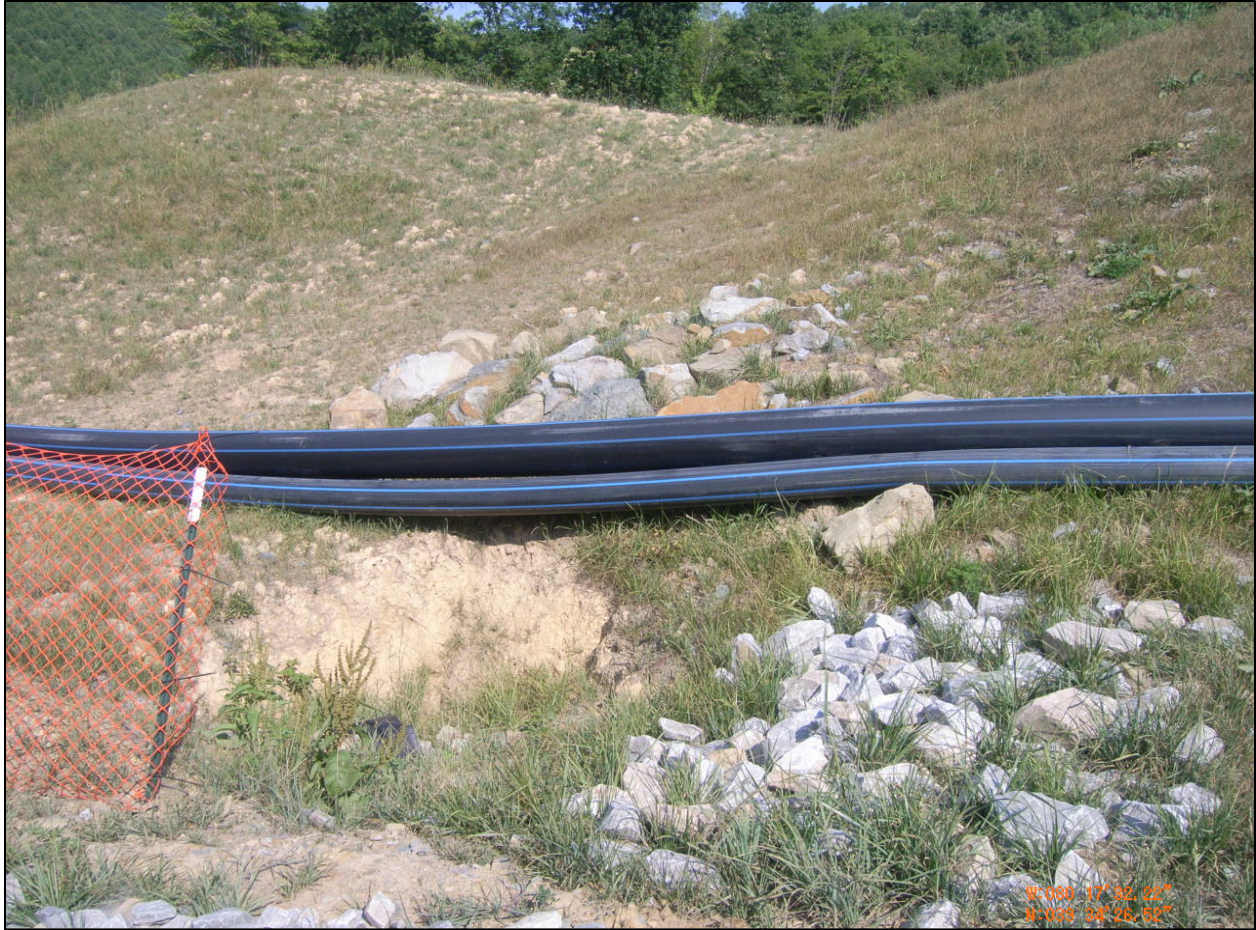
Figure 10: Unsupported Pipe
