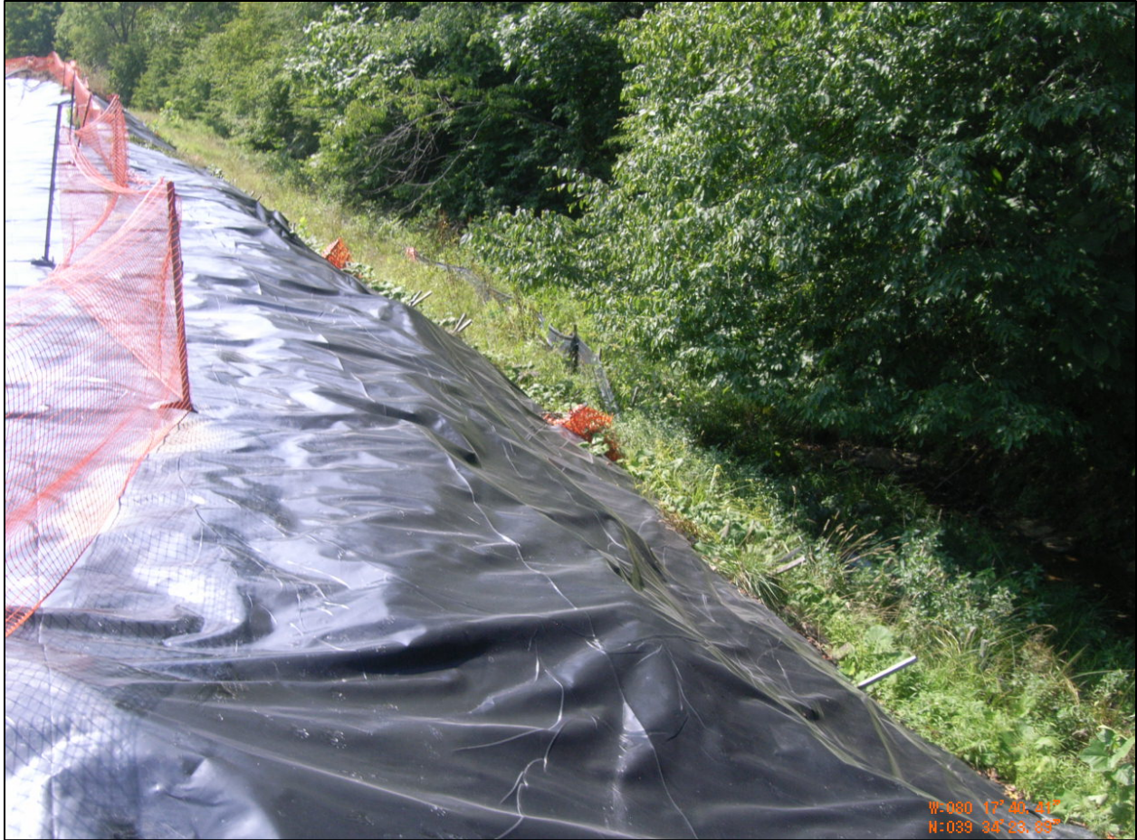
Figure 5: Bulges on Downstream Face
