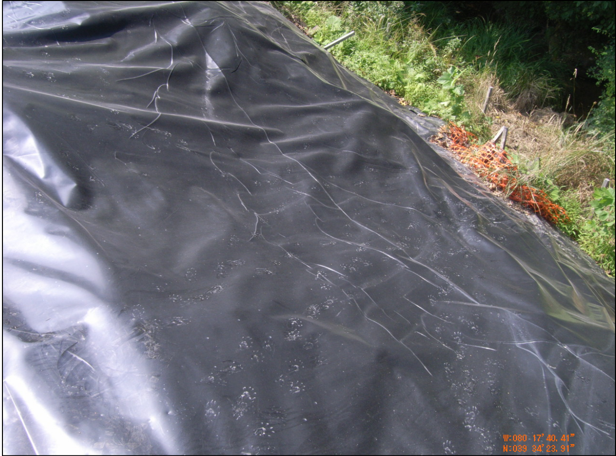
Figure 11: Downstream Slope Movement into Ditch
