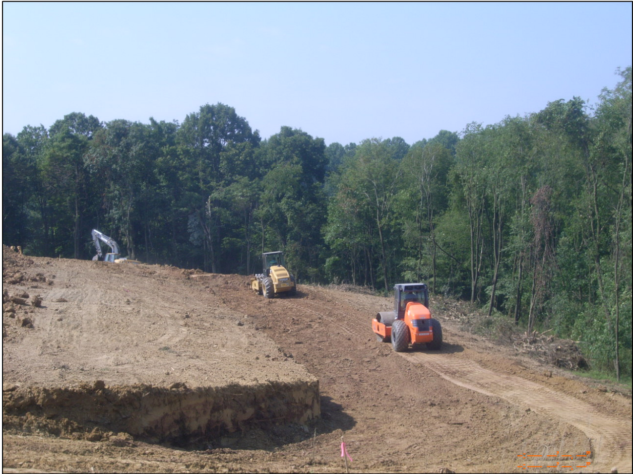
Figure 20: Improper Compaction Practices
