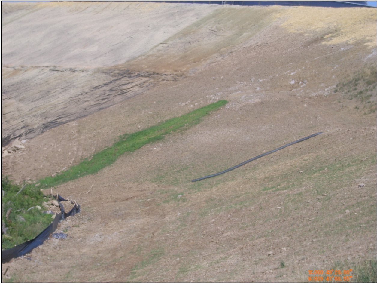
Figure 15: Seepage at Pribble
