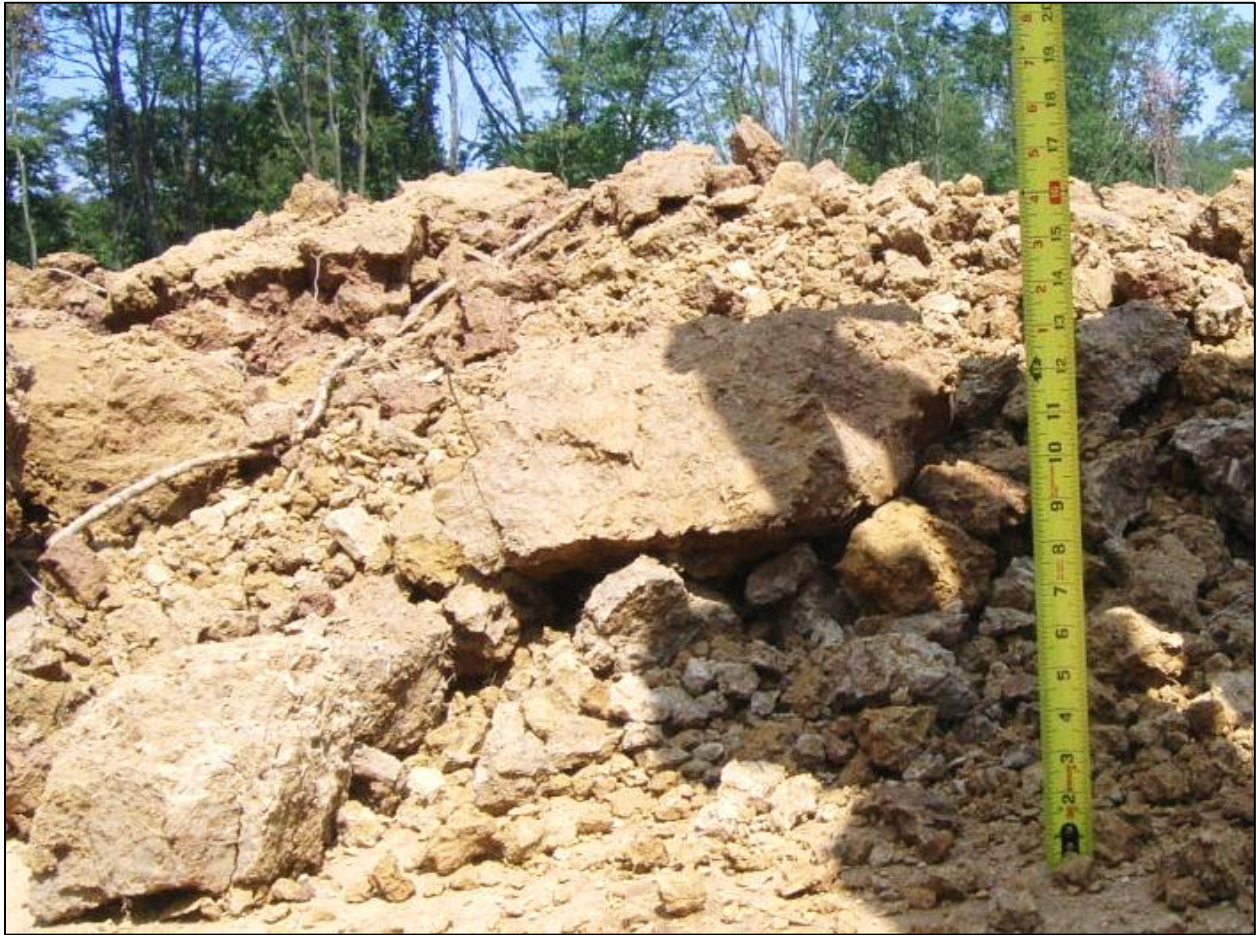
Figure 22: Excessive Lift Thickness
