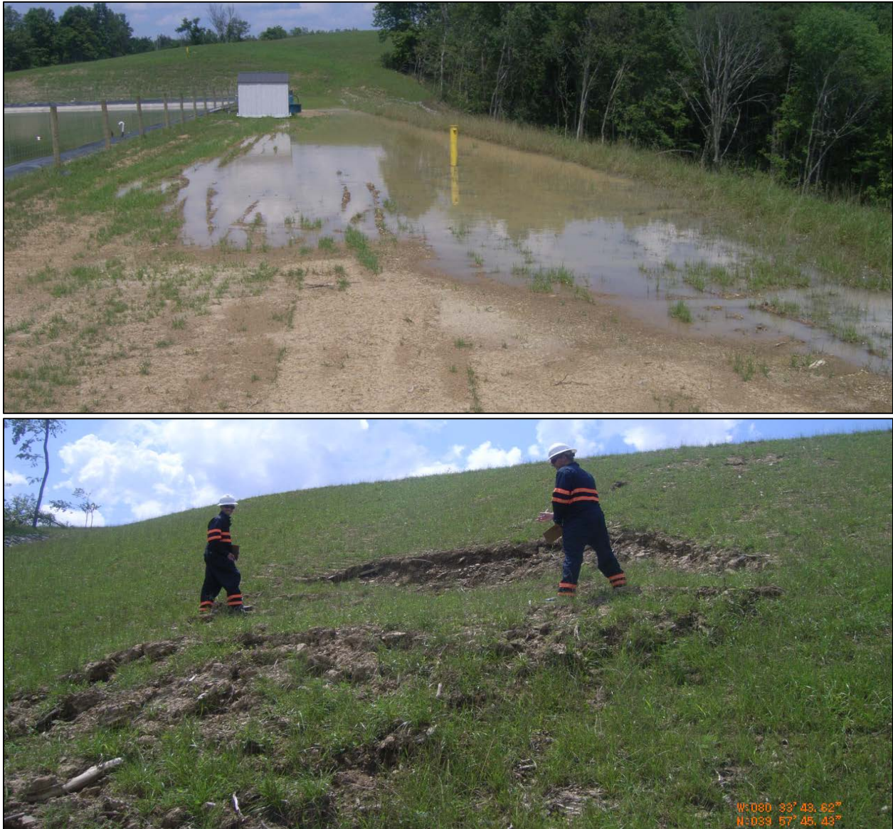
Figure 13: Slope Movement at SHL 4
