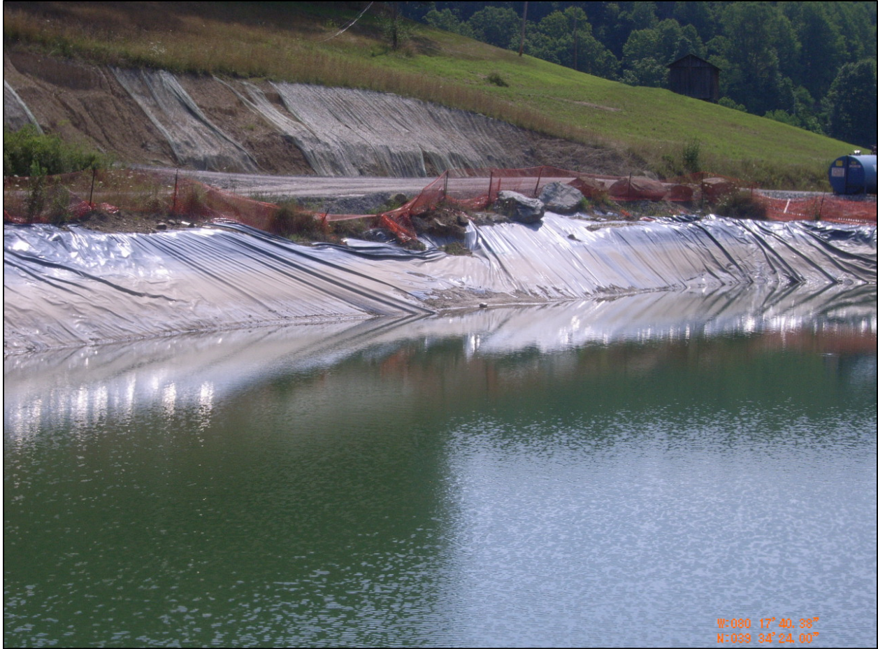
Figure 6: Slope Movement into Impoundment
