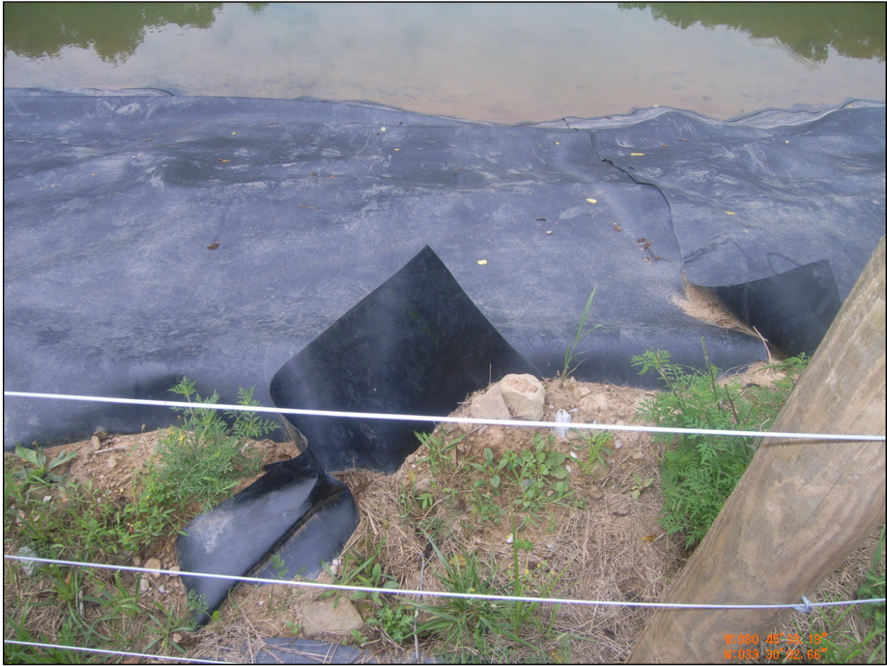
Figure 18: Improper Anchor Trench Embedment at Ball 1H
