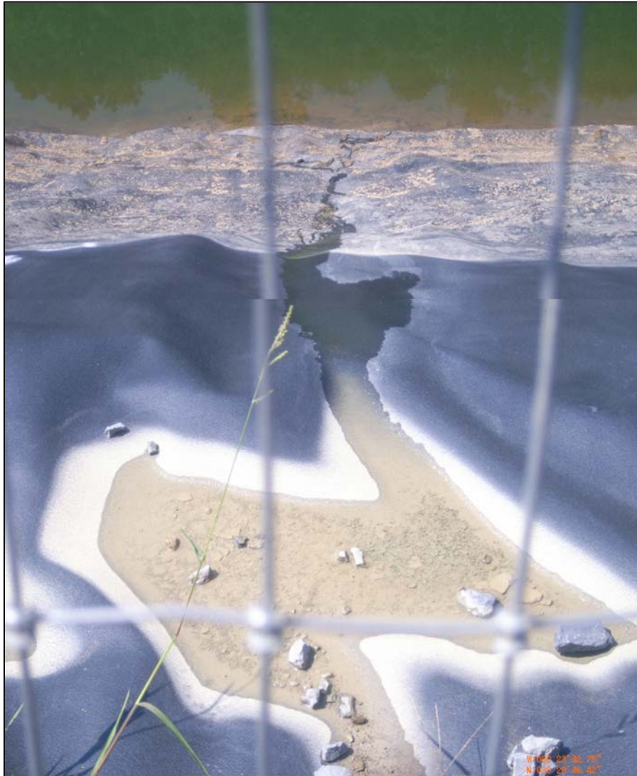
Figure 17: Debris on Liner at Flanigan
