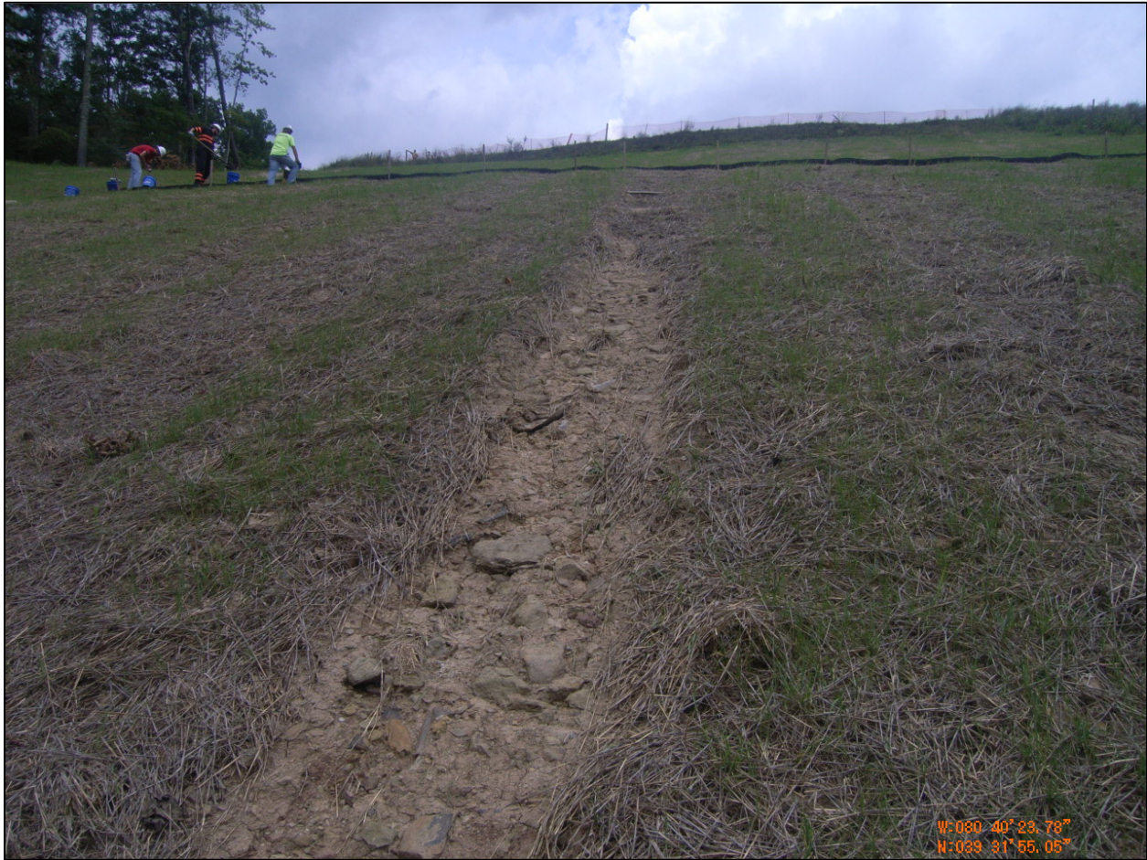
Figure 12: Surface Erosion at Mills-Wetzel
