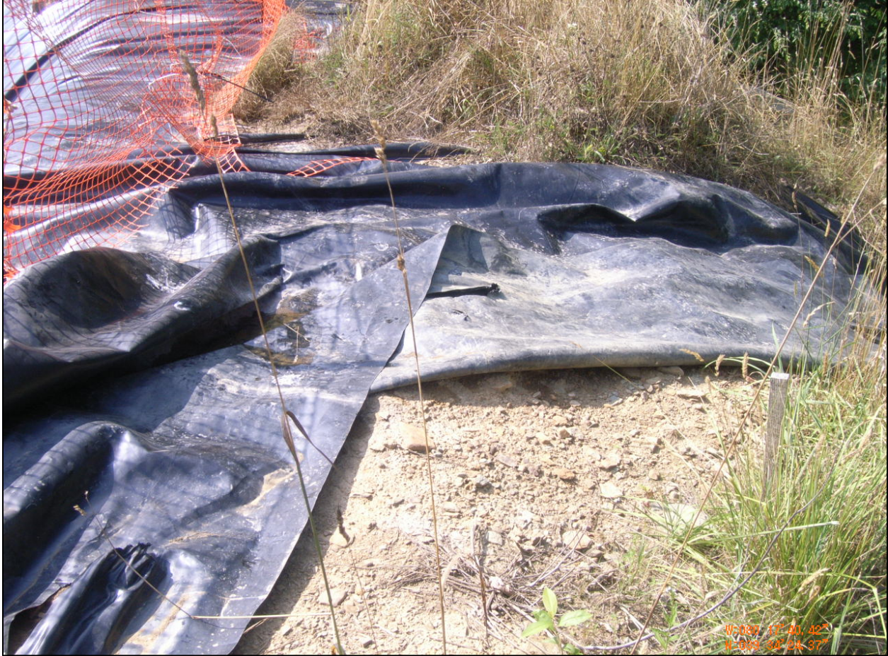
Figure 9: Anchor Trench Exposed
